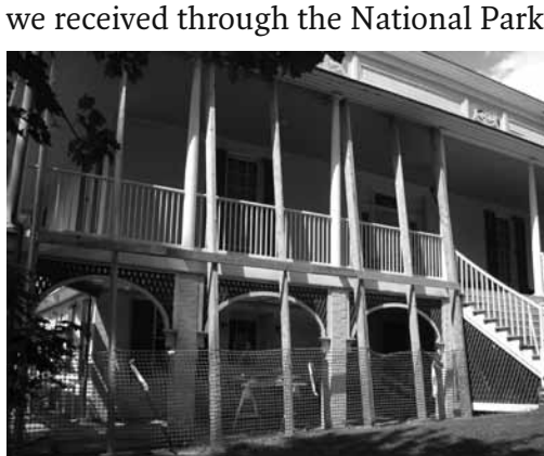
Construction work on the Main House
